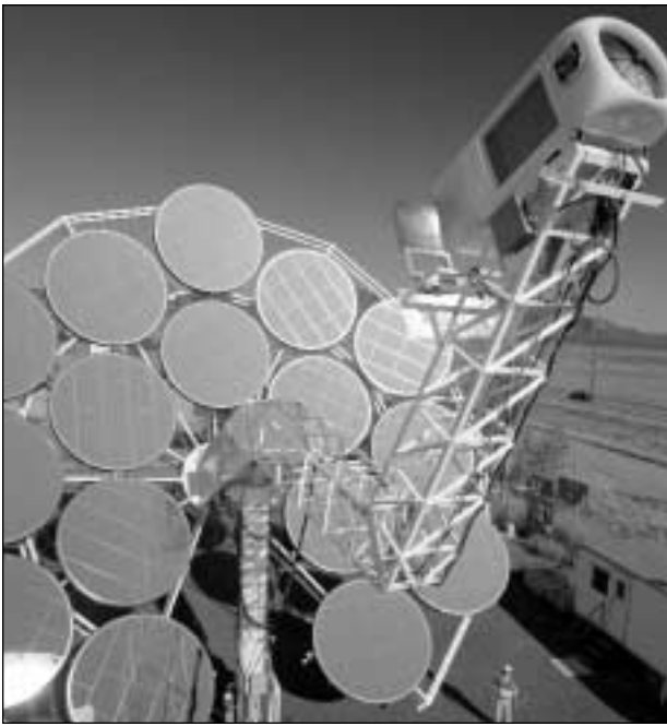
This concentrating solar power system uses mirrors to focus highly concentrated sunlight onto a receiver that converts the sun's heat into energy.
